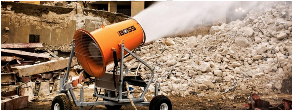
Atomised mist sprayed over work area to reduce dust.
